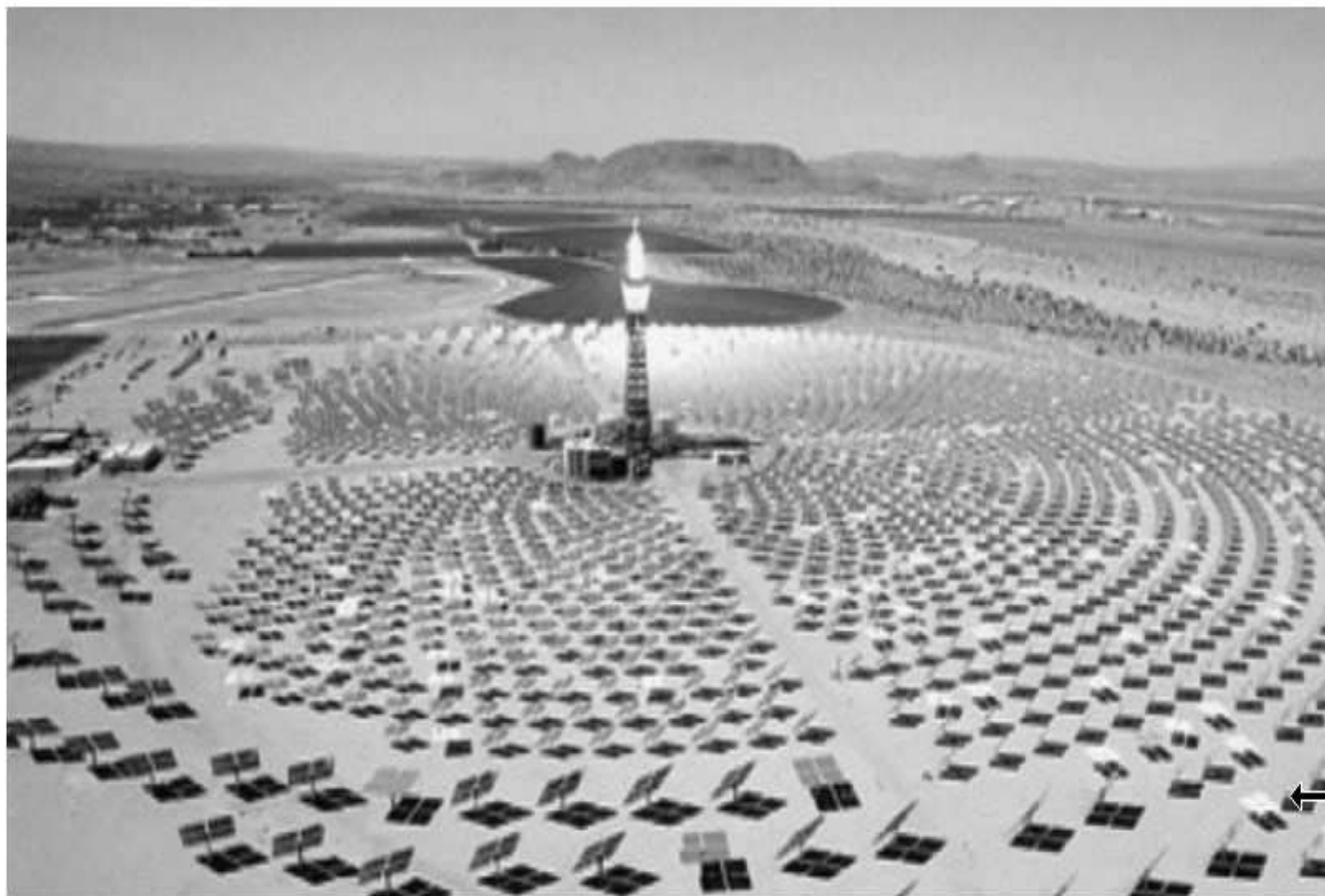
Photograph of the Solar Two central receiver plant
